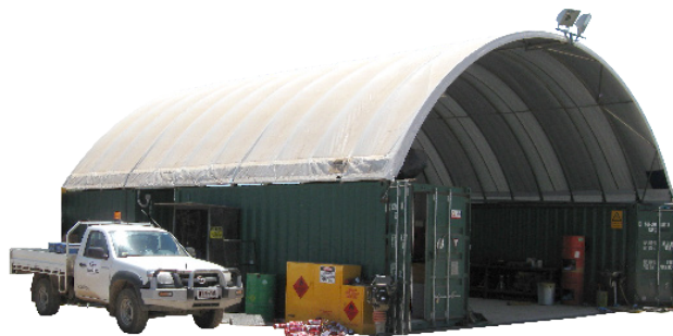
Example of a Shipping Container Shelter
